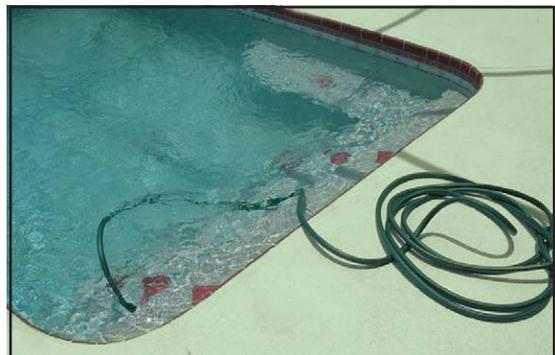
*Submerging a hose in a swimming pool could create a potential backflow hazard*
